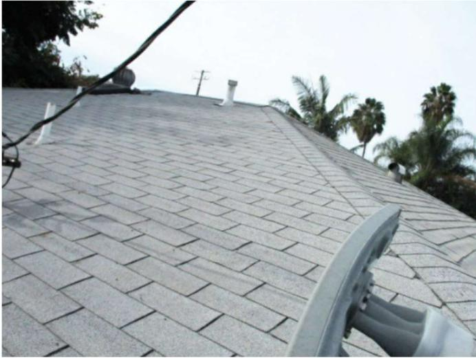
On some older homes, you might even notice three or four layers of shingles placed atop each other, when there should only be one. This indicates past attempts at patching rather than removing and completely replacing the roof.
